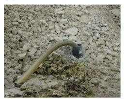
The entire area is isolated from the subgrade by a geotextile membrane then by a geomembrane and is equipped with a drainage network and a degassing vent system. The latter system consists of a honeycomb structure placed underneath the lower geomembrane.
