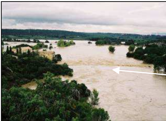
The Saint-Nicolas bridge in Uzès (Gard), submerged by flood waters - 09/09/2002
