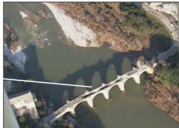
View of the bridge 5 days later
