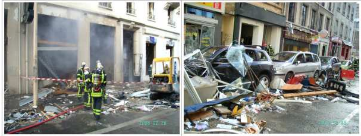
Property damage - Source: DREAL (Regional Environmental Agency) Rhône-Alpes
